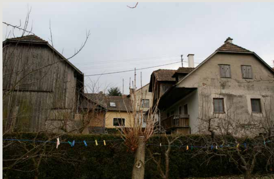
Garden view prior to renovation
